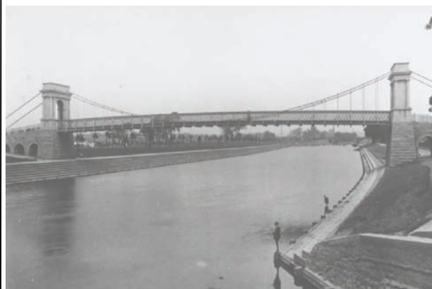
WEST BRIDGFORD SUSPENSION BRIDGE
